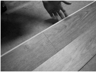
Fig. 6 - Locking long side with ends already locked
