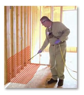
The 2-foot band treatment is needed to protect the structure from termites. This gives termite and general pest protection at the base of walls where pests tend to build nests if they get access to a home. Bora-Care also protects against entry over treated concrete and around plumbing penetrations.
