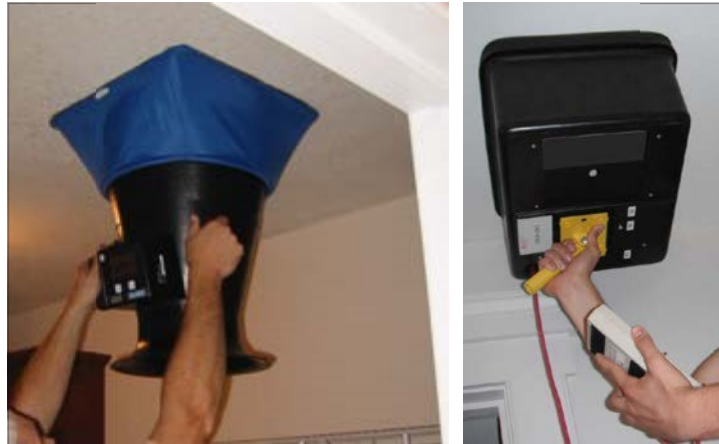
Figure 8. Measuring Exhaust Flow with a Flow Hood and Exhaust Fan Meter.
